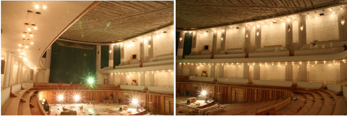
Figure 5.- Construction progress January 2007
