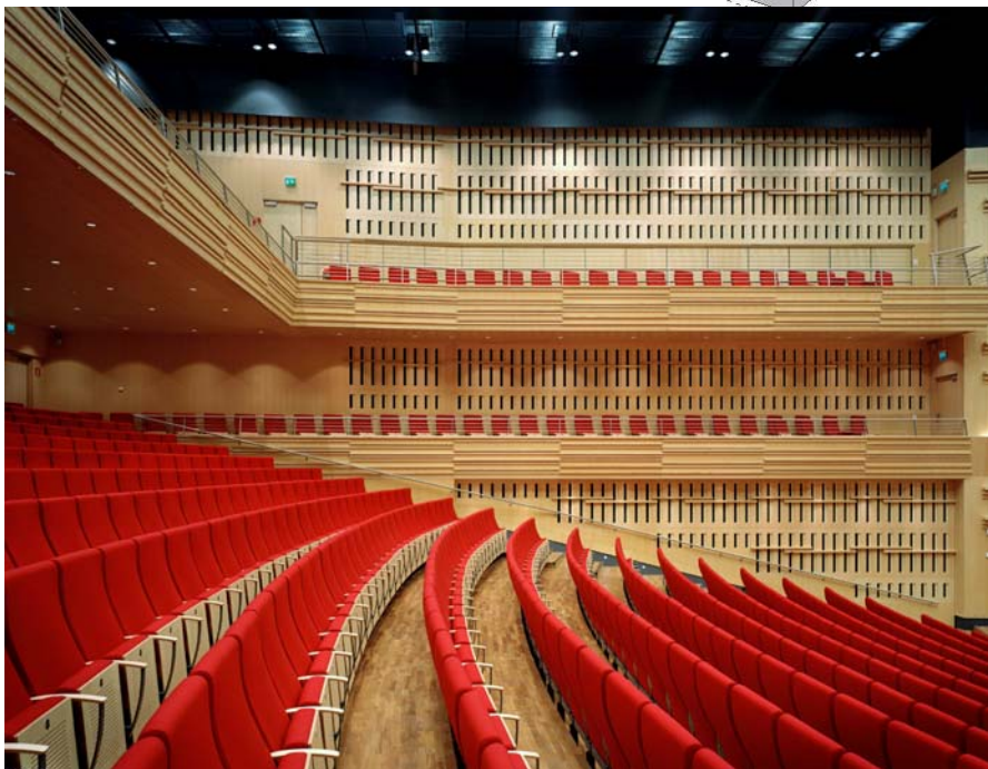
Figure 1. – Lulea House of culture a) Exterior b) CATT model c) Interior side walls with adjustable wall panel absorbers. The wall panels are shown in opened condition. Black squares are mineral wool absorbers.
