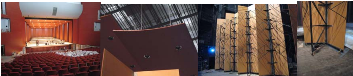
Figure 3.-The orchestra shell, a ceiling panel, light structure, wheel system
