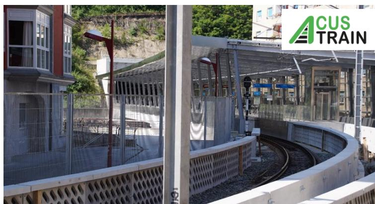
Figure 5 – Image of the Acustrain™ Low Noise Barrier installed at Ermua.
