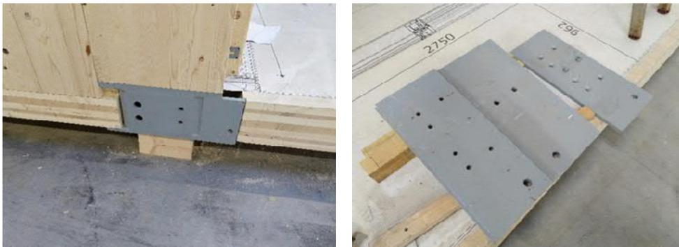
Figure 4. The floor steel element (left) and the steel connection plates (right).
