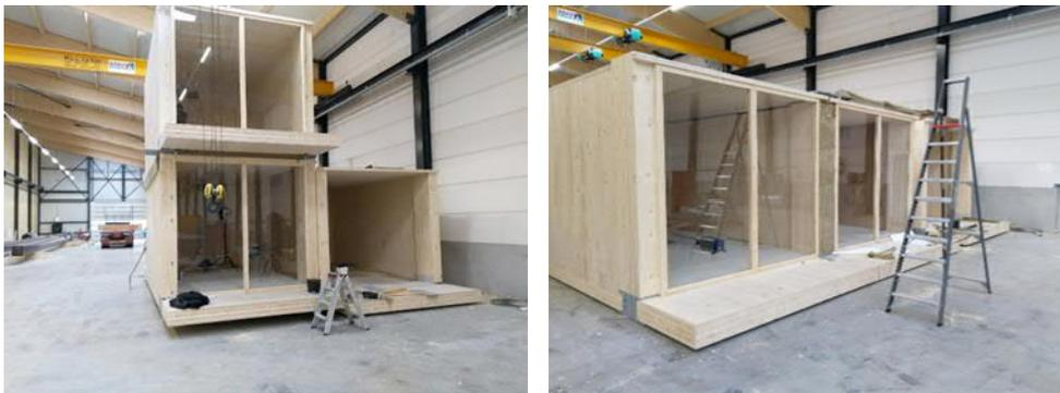
Figure 3. The CLT modules in the vertical arrangement (left) and in the horizontal arrangement (right).
