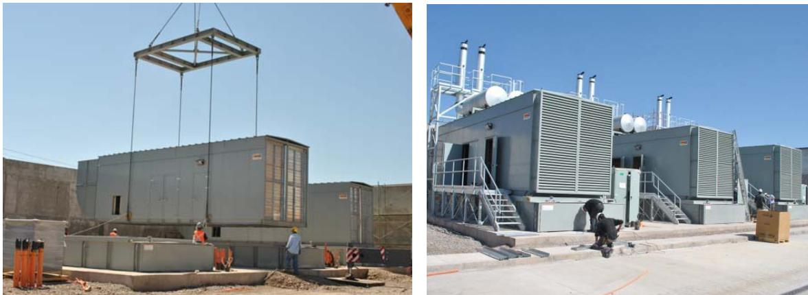
Figure 7 – HP Data Center Enclosure. b) enclosure being installed, c) enclosure finished.
