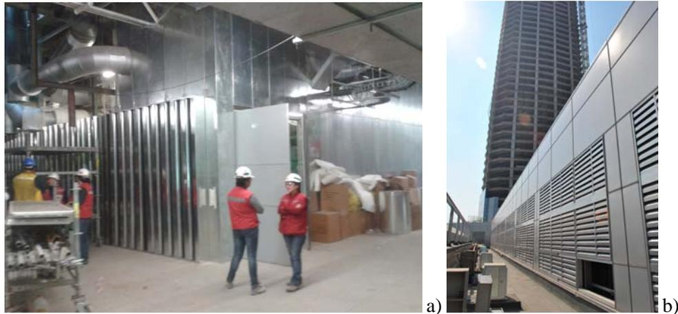
Figure 9 – Costanera Center Mechanical room, a) Power Generation room, b) acoustic louvers.
