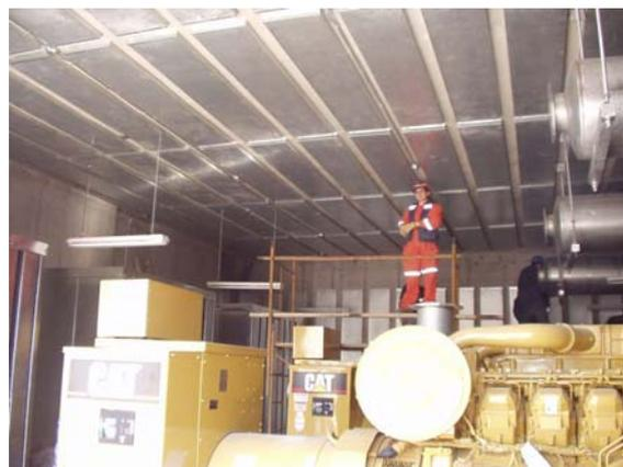
Figure 1 – a) Isolating and sound absorbing wall, b) Sound absorbing panels
