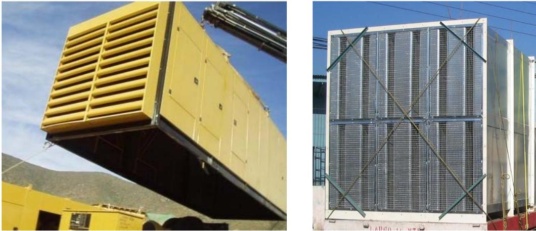
Figure 2 – Inlet and outlet silencers. a) Acoustic louver b) rectangular silencer.
