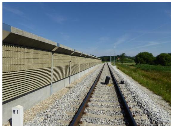
Figure 2 – The photos of the investigated barrier configurations – flat absorptive finishing and T-finishing
