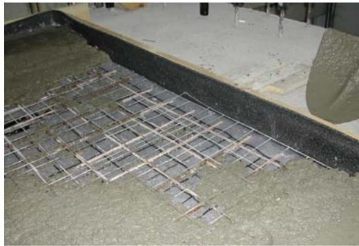
Figure 2 - Final concrete layer of the floating floor.
