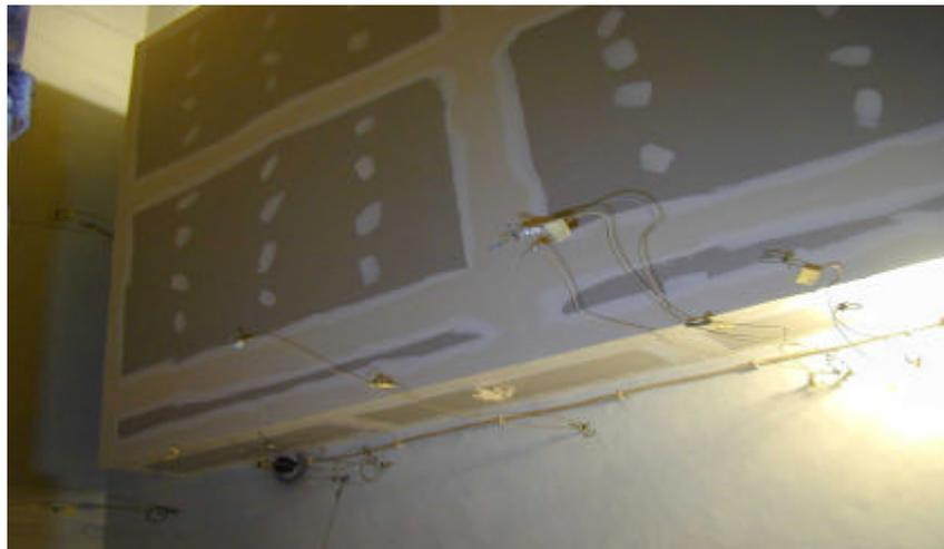
Fig. 1 – Overview of a false ceiling constructed in the test room
