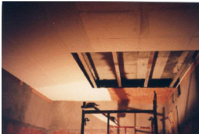
The first picture shows the experimental patchwork built to demonstrate that a uniform surface can in fact hide several components, some reflective, some absorptive.
