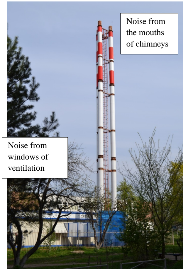
Fig.1 Boiler house with medium power boilers
