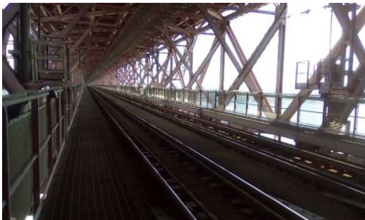
Figure 2 – Barriers installed at the rail platform
