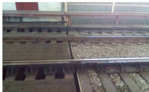
Figure 3 – Detail of the transition zone between the suspended bridge and the access viaduct
