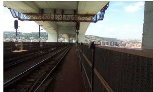
Figure 2 – Barriers installed at the rail platform
