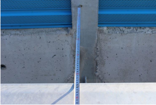
Photo 8 Distance between the restraining system and the noise barrier – 37.5cm
