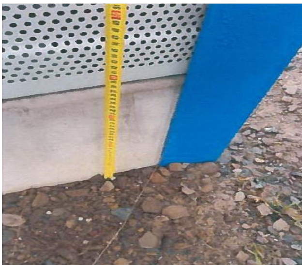
Photo 3 Continues concrete footing – 50cm
