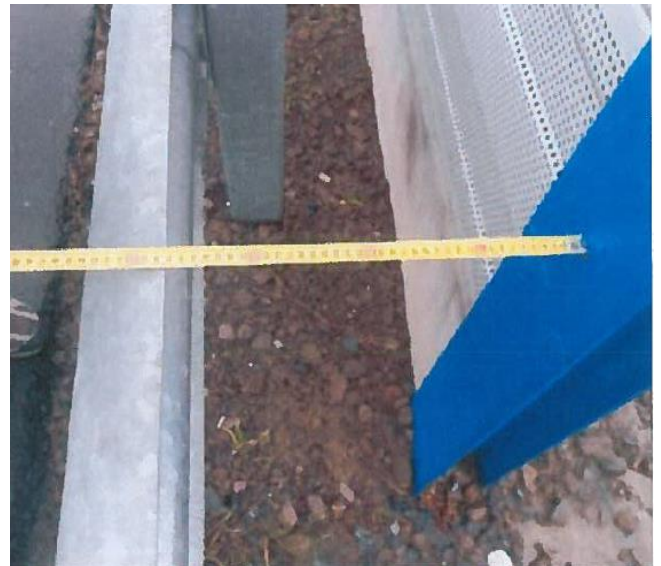
Photo 2 Distance between the restraining system and the noise barrier – 37.5cm
