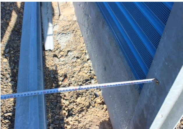
Photo 11 Distance between the restraining system and the noise barrier – 40 cm
