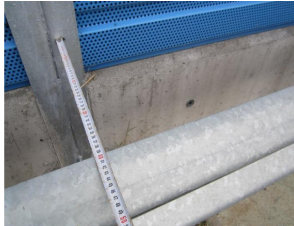
Photo 12 Distance between the restraining system and the noise barrier – 40 cm
