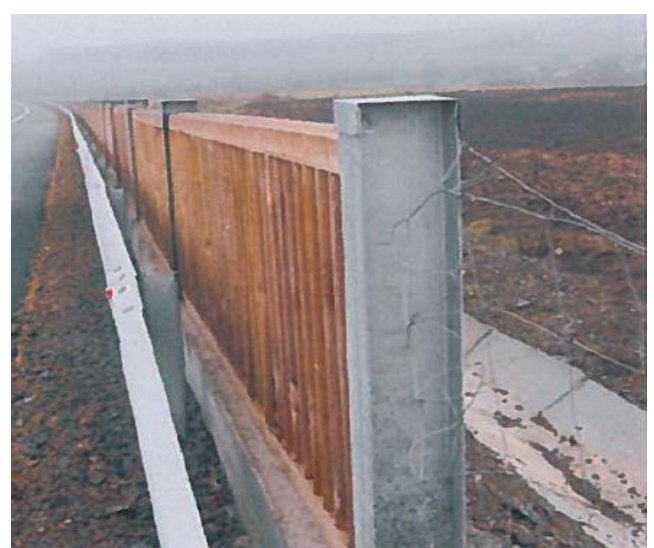
Photo 4 Wooden noise barrier
