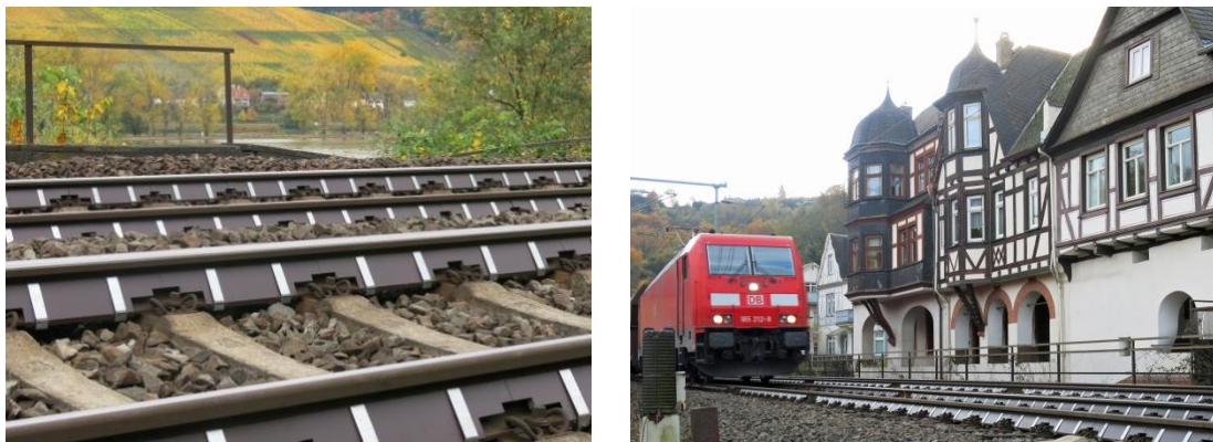
Fig.6: RWS – boltless Calmmoon Rail on DB AG track in the Rhine Valley
