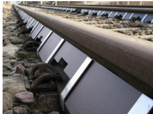
Fig.2: Calmmoon Rail on UIC 60 rail
