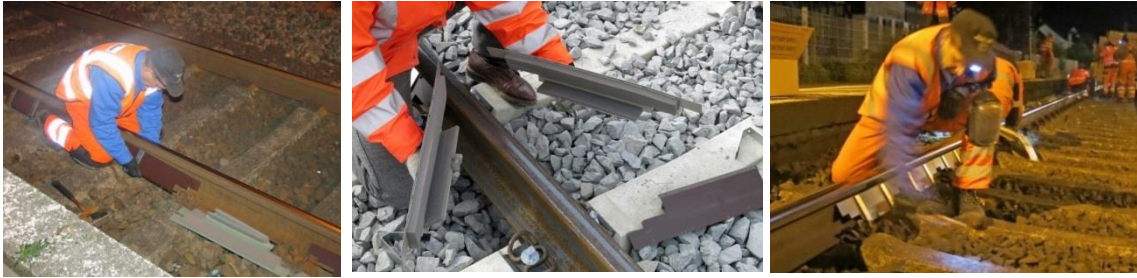
Fig.5: Fitting Calmmoon Rail web shielding
