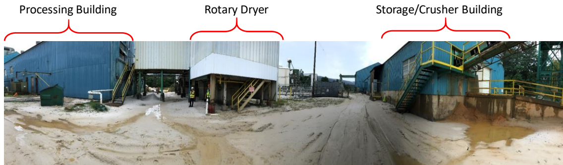
Figure 10: Area outside the processing building, rotary dryer, and storage/crushing building.
