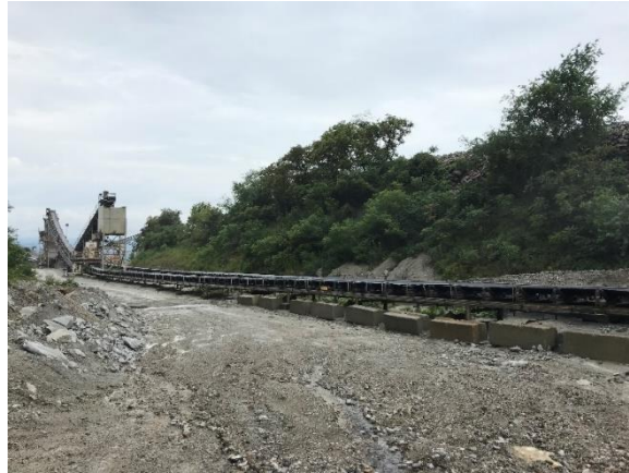
Figure 12: Primary conveyor with primary screen in far distance.
