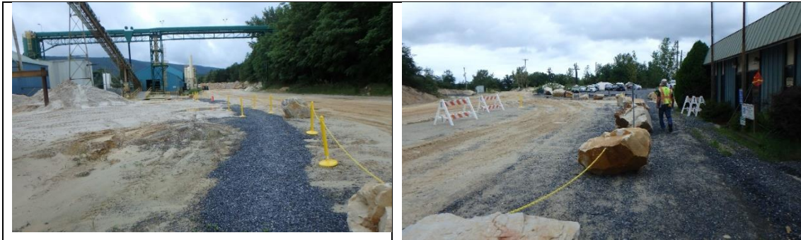
Figure 17 B: Pedestrian walkway installed
