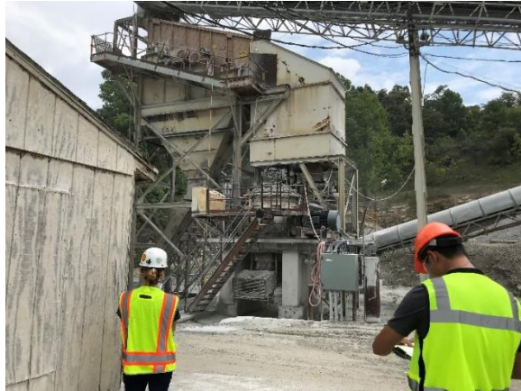
Figure 14: Outside area near the secondary crusher/screener
