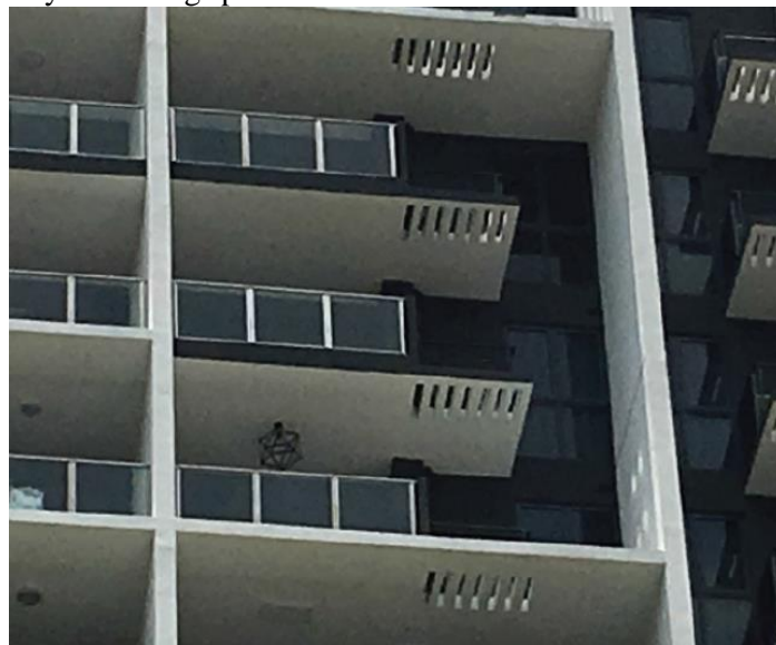
Figure 8: Glass barrier at balcony in residential development
