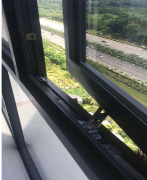
Figure 7: Window restrictor on the windows
