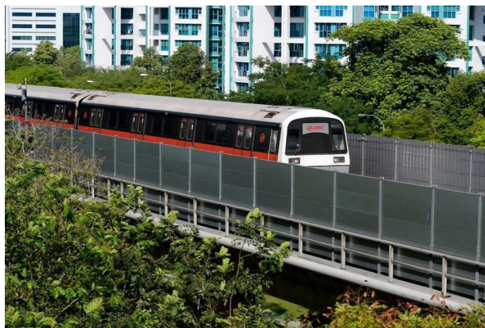
Figure 1: Noise Barriers at above ground MRT track
