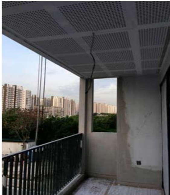
Figure 6: Acoustic ceilings on balconies in residential development
