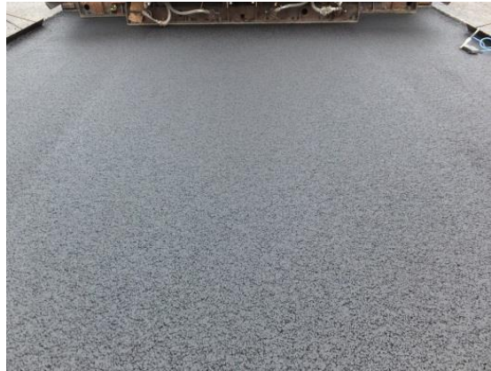
Photograph 2 - Example of road-laying using a general AF
