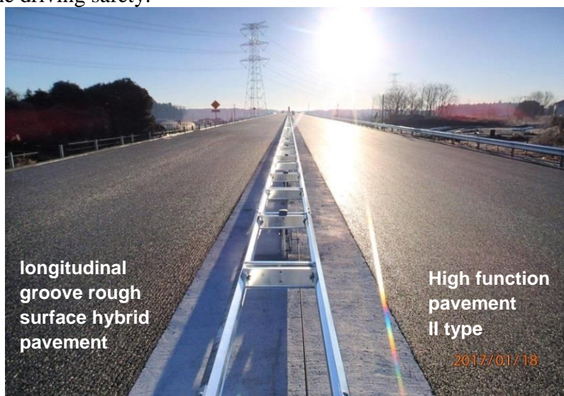
Photograph 4- Example of improving visibility by limiting the diffuse reflection of sunlight
