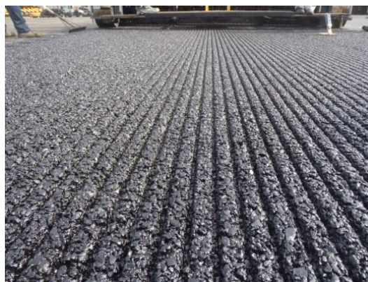
Photograph 1 - Example of longitudinal groove rough surface finishing
