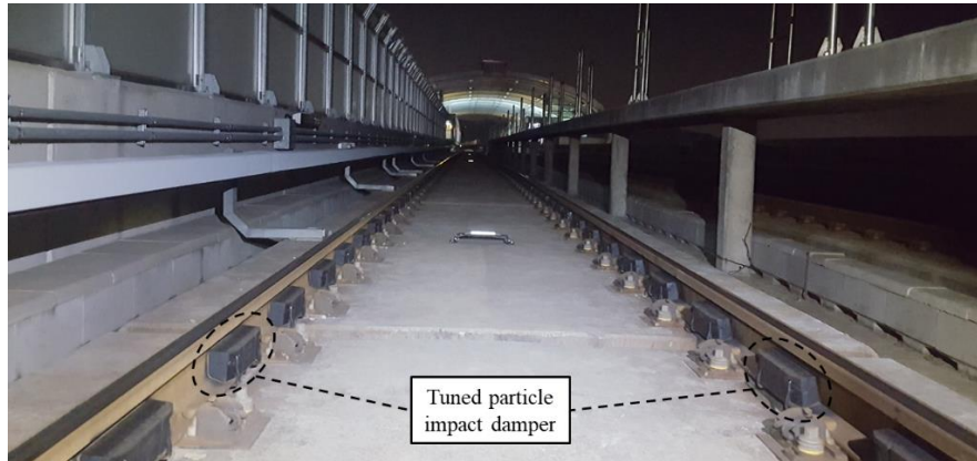
Figure 1. Tuned particle impact dampers on actual track
