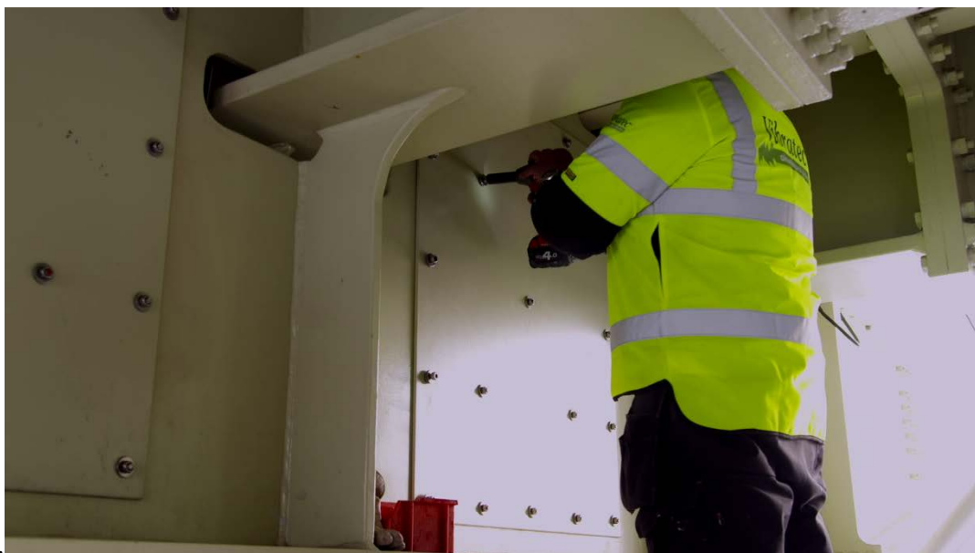
Figure 3. Mounting of CLD element onto transverse plate.
