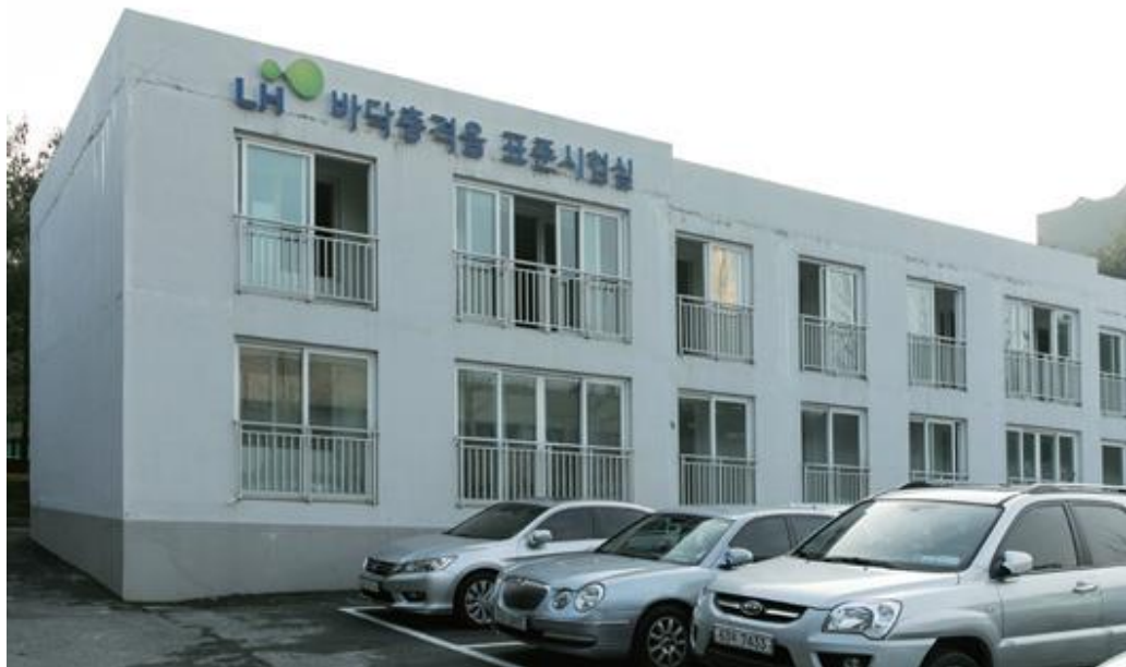
Figure 2 – Standard Testing Laboratory for Floor Impact Noise in Korea
