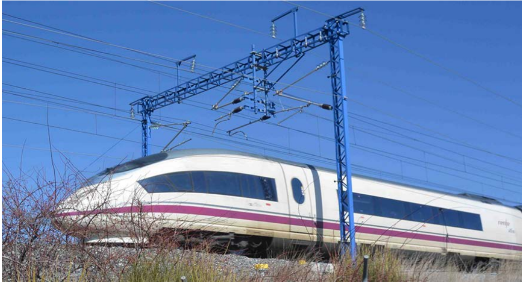
Figure 3.1.2: Pass-by of a RENFE series 103 under the instrumented catenary portal.
