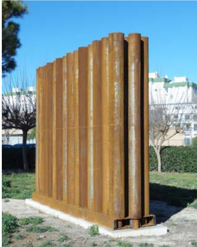
Figure 5. Noise barrier based on sonic crystals.
