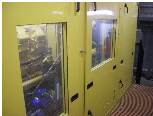
Figure 5: Engine enclosure highlighting observation and inspection windows
