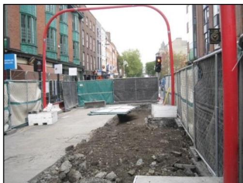
Photographs 3-4 Acoustic blankets installed on Marlborough Street (left) and Hawkins Street (right)
