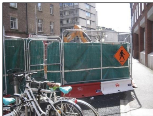
Photographs 3-4 Acoustic blankets installed on Marlborough Street (left) and Hawkins Street (right)
