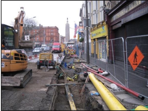
Photographs 1-2 Utility diversions on Marlborough Street (left) Rail installation on Nassau Street (right)
