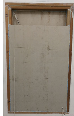
Figure 2: Front view of a tested ventilation partition from the receiver room.
