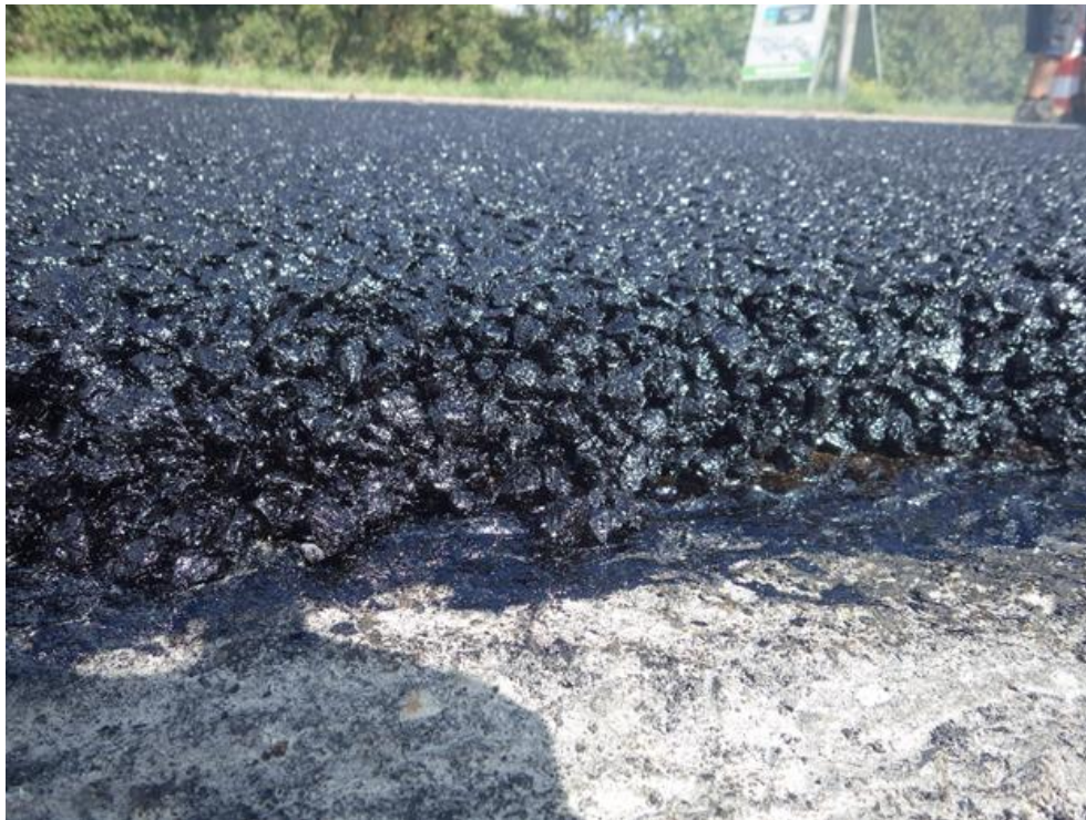
Figure 4 Porous asphalt layer
