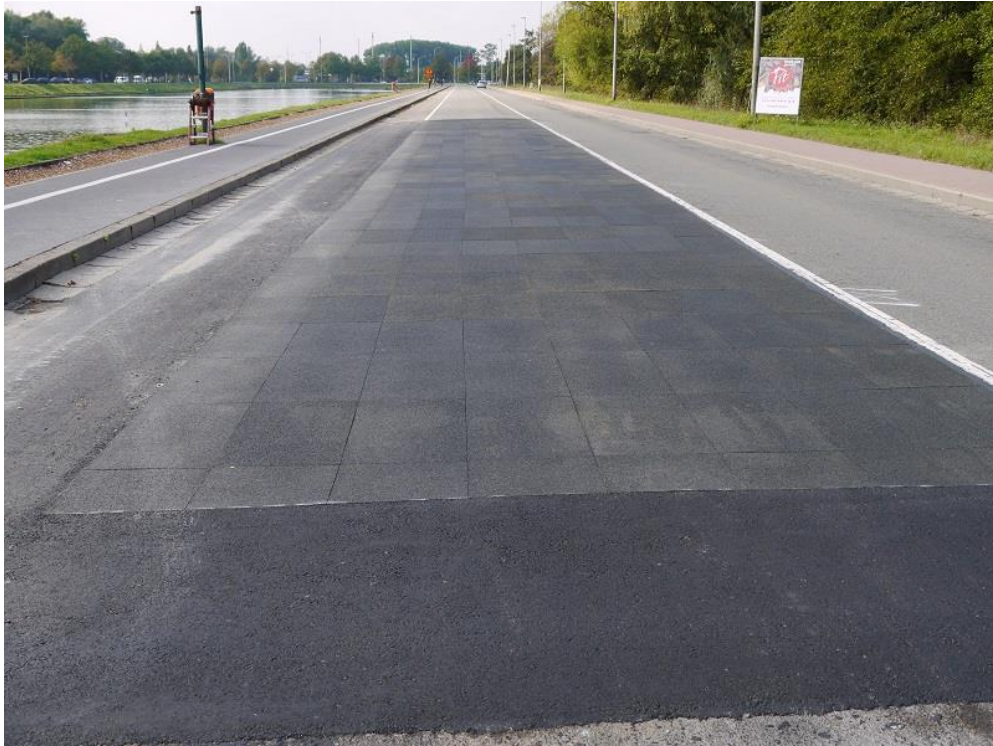
Figure 8 View on the PERS test track one day after opening for the traffic
