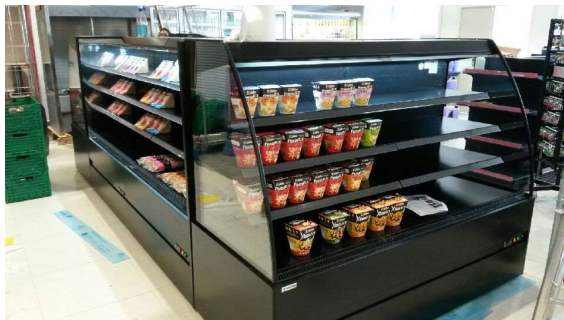
Figure 8: indoor unit in the shop area (display case) [3]
