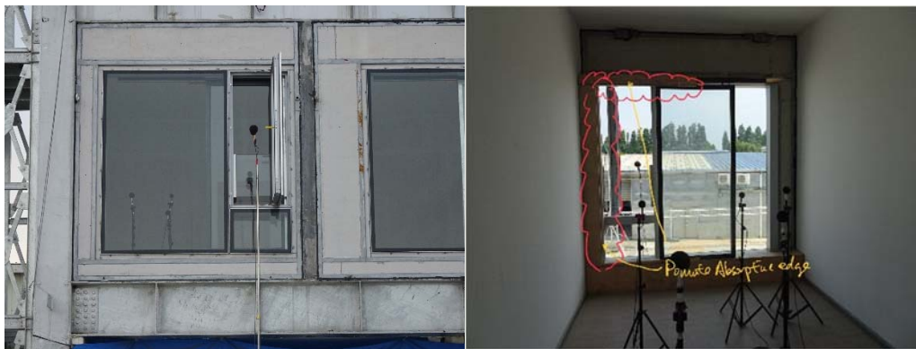
Figure 4. Microphones setup (left: facade; right: indoor) and the locations of the installed absorption
