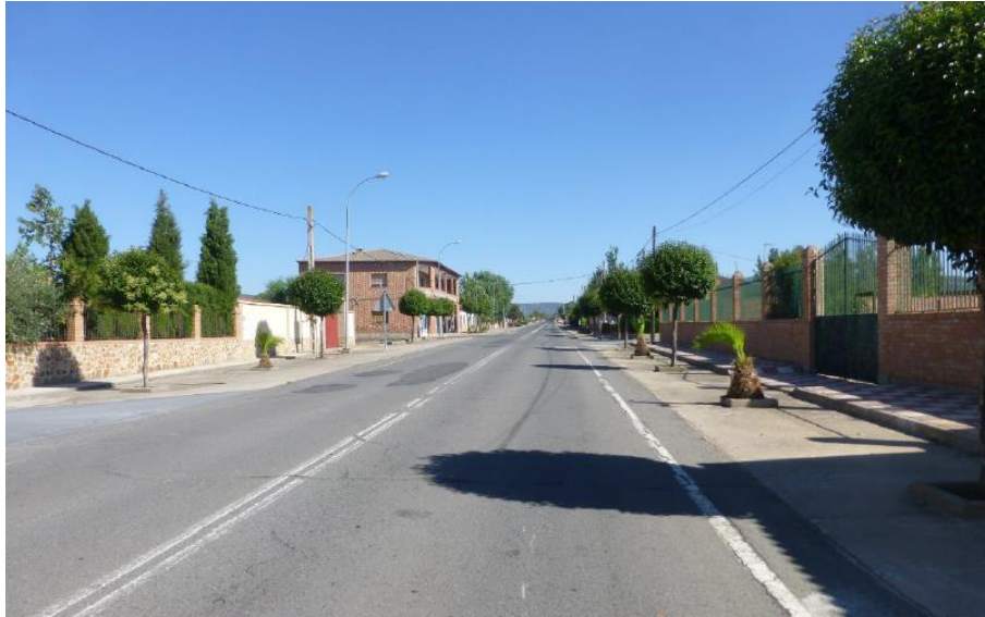
Figure 2: Experimental section AC22 before rehabilitation with the Cold-In place-Recycled pavement.
