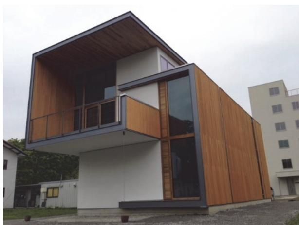
Fig. 1 – Photograph showing the outside view of CLT model building.
