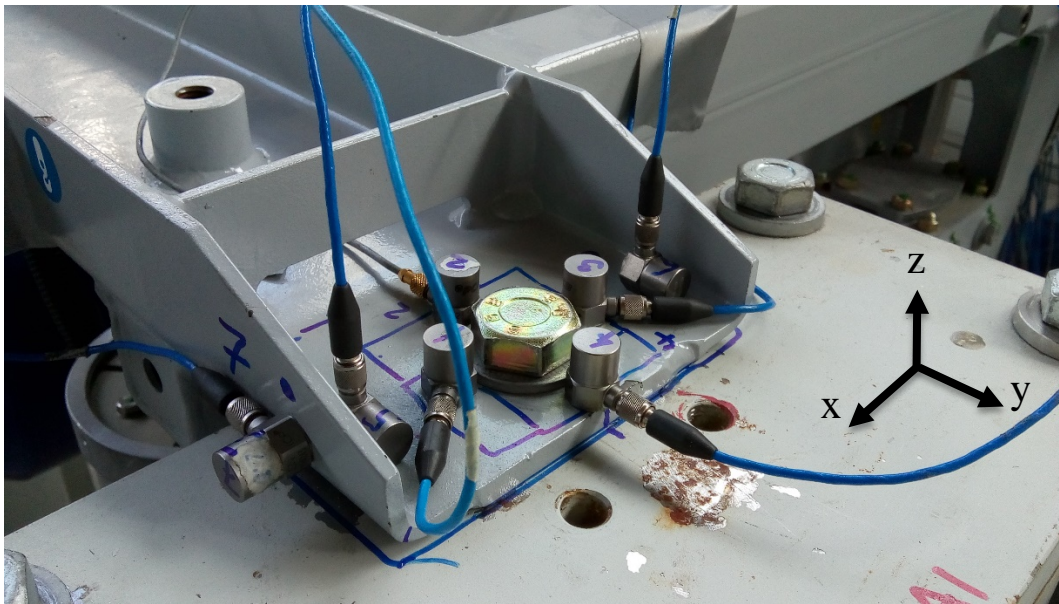
Fig. 2 – Instrumentation of AGTU connection point
