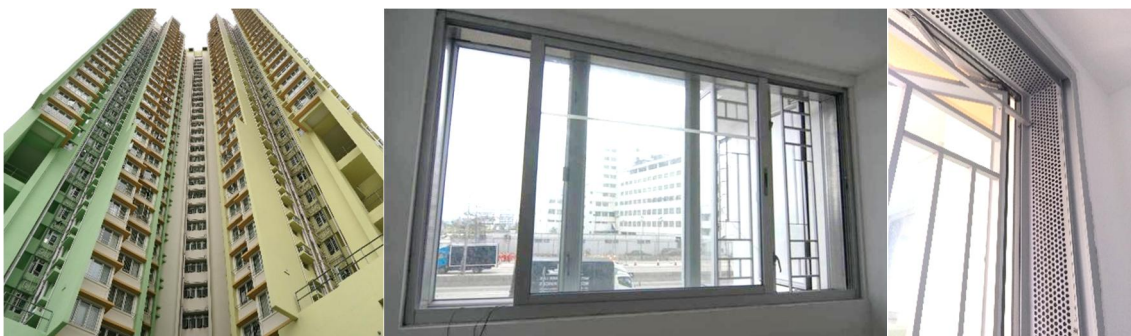
Figure 4 – Acoustic window in King Tai Court, San Po Kong
