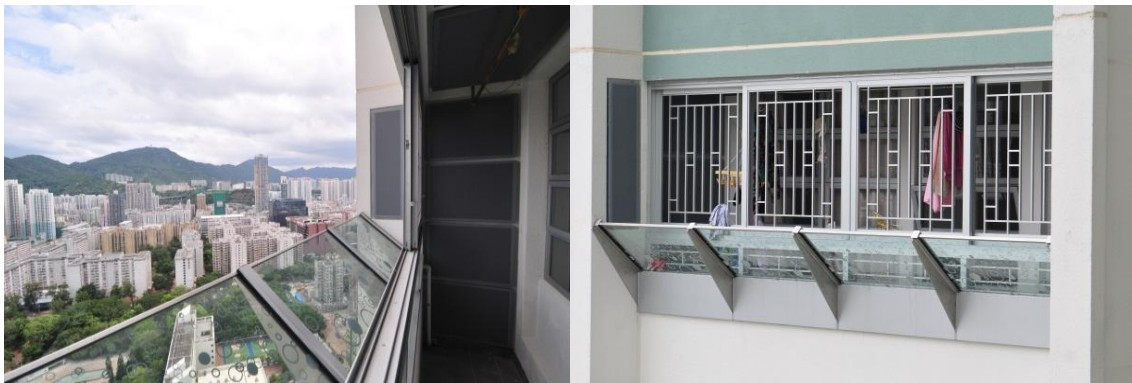
Figure 9 – Acoustic balcony in Wing Cheong Estate, Sham Shui Po
