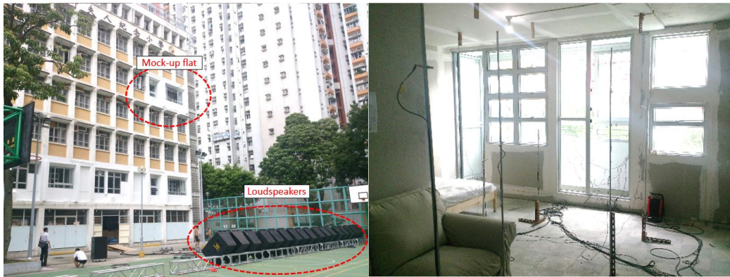
Figure 11 – Mock-up test in Wing Tai Road, Chai Wan
