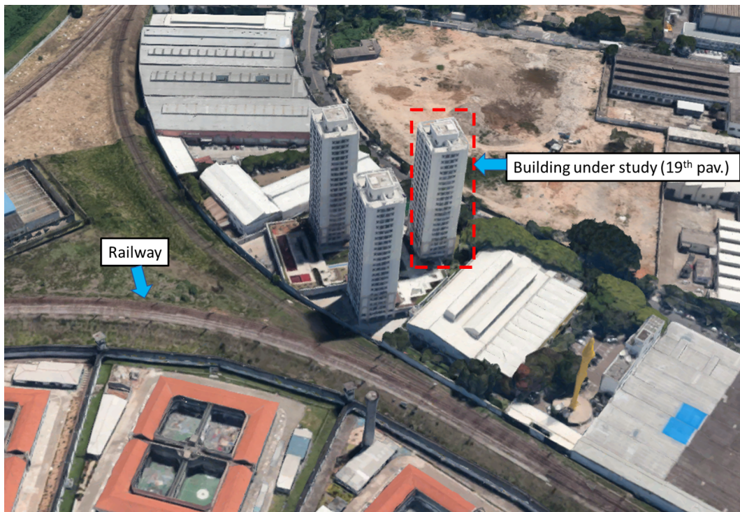
Figure 1: Location of the building and the railway
