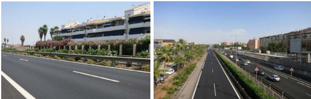
Figure 10. (a) Image of the road A8058 after paving mixtures. (b) The same at A-376.
