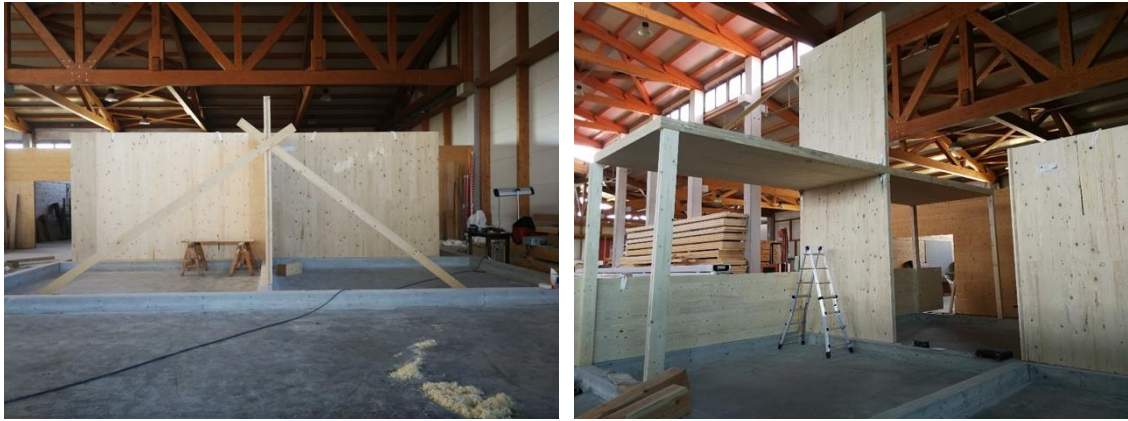
Figure 1: Pictures from the setup: “X” vertical junction (left) and “X” horizontal junction (right).
