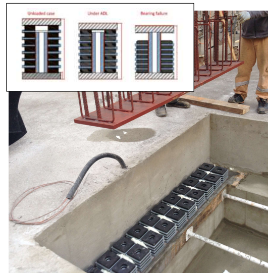
Figure 11. Installation of the VHS (very high stress) bearings with integrated failsafes.
